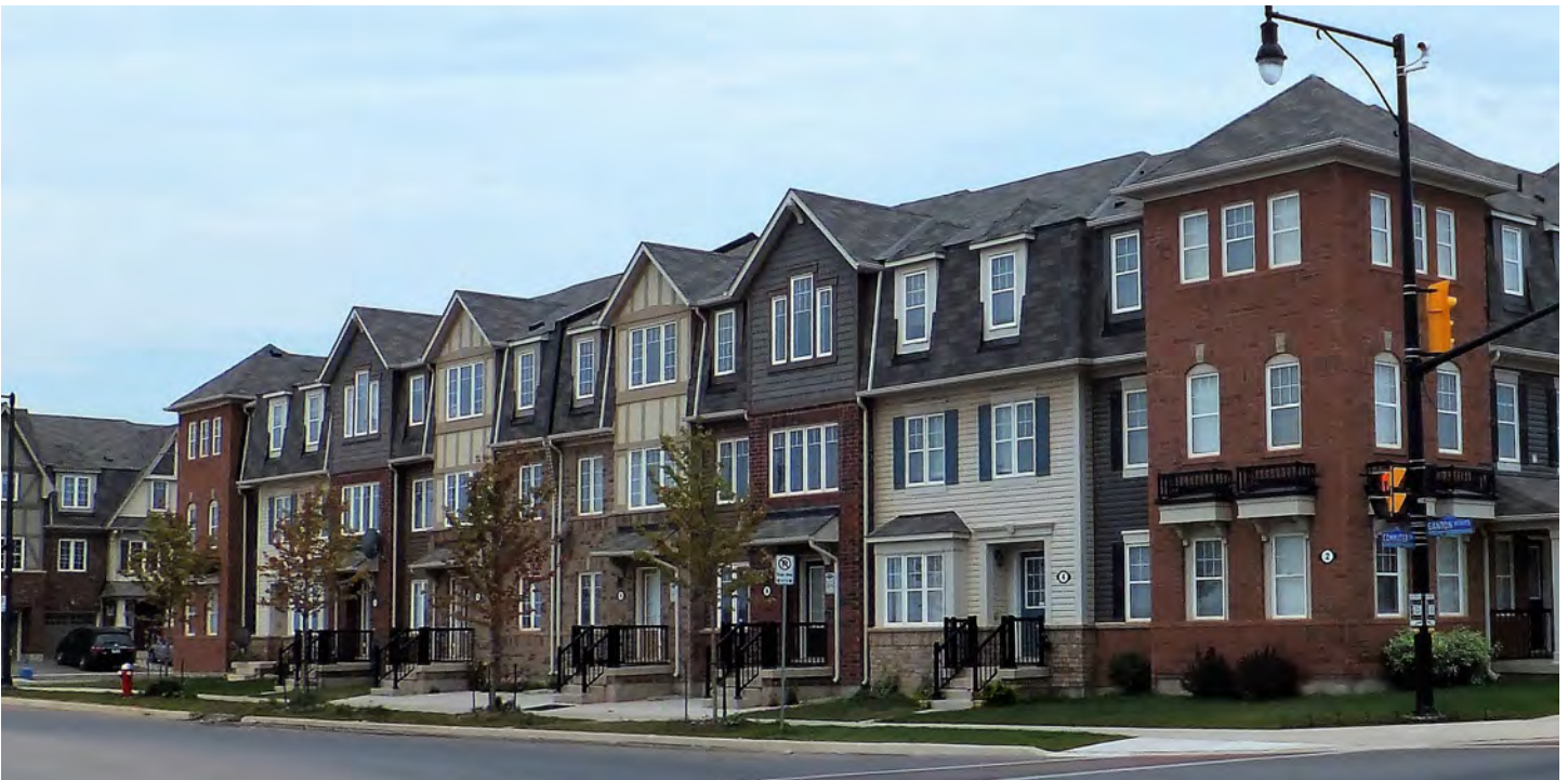
Variety in housing options. Medium density housing in the form of townhouses.
