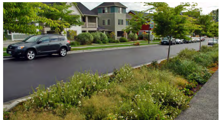
A bioswale in the right-of-way to assist with run-off and infiltration.
