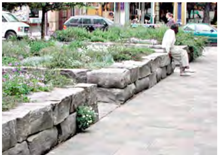
Light coloured pavers assist with the reduction of the urban heat island effect.
