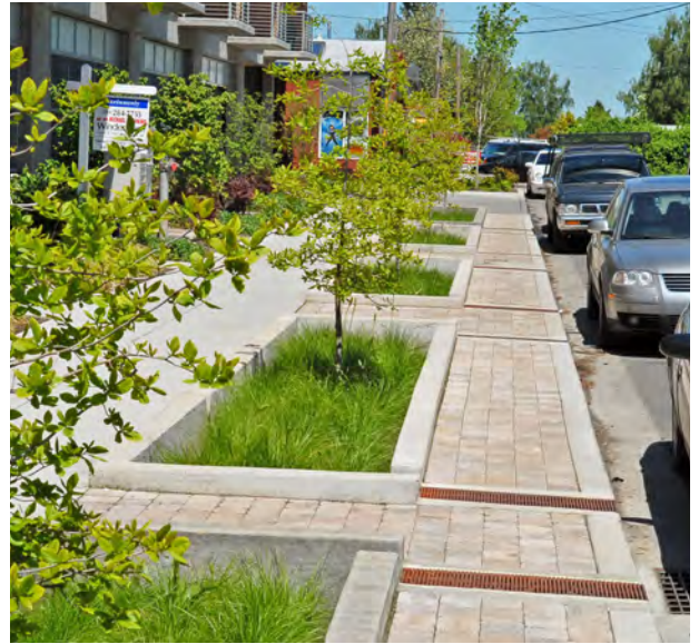
Bioretention planters have stormwater management benefit.
