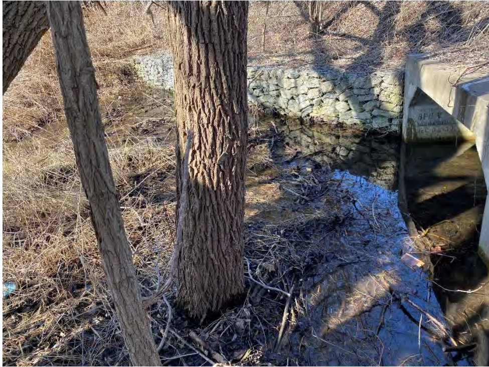
George Reynolds Drive Culvert South Side (downstream outlet)
