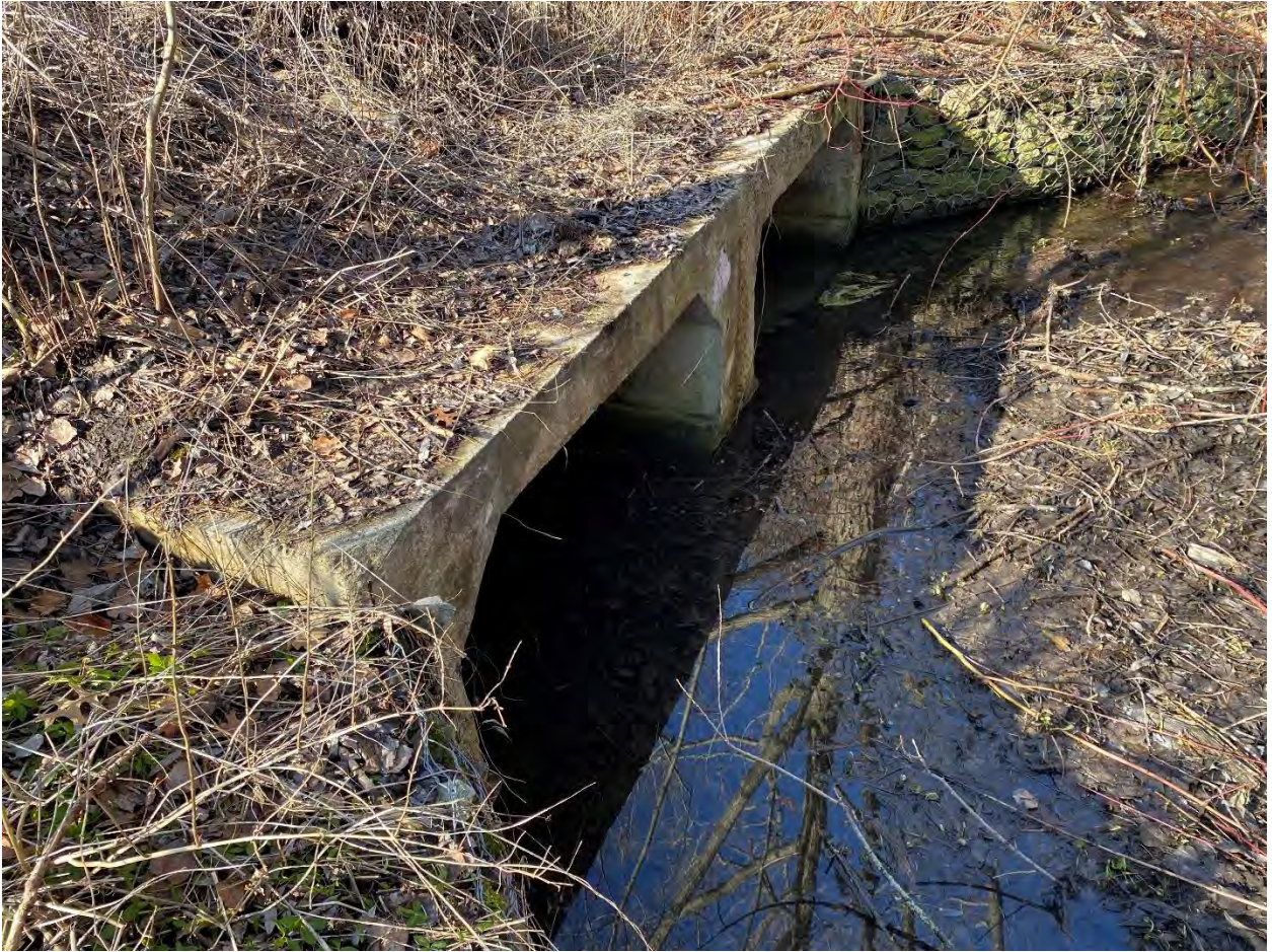
George Reynolds Drive Culvert North Side (upstream inlet)
