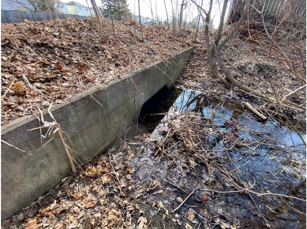
Trulls Road Culvert West Side (downstream outlet)
