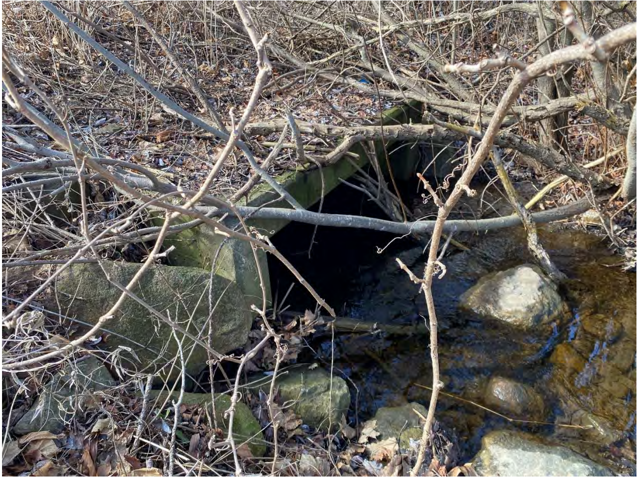
Devondale Street Culvert North Side (upstream inlet)
