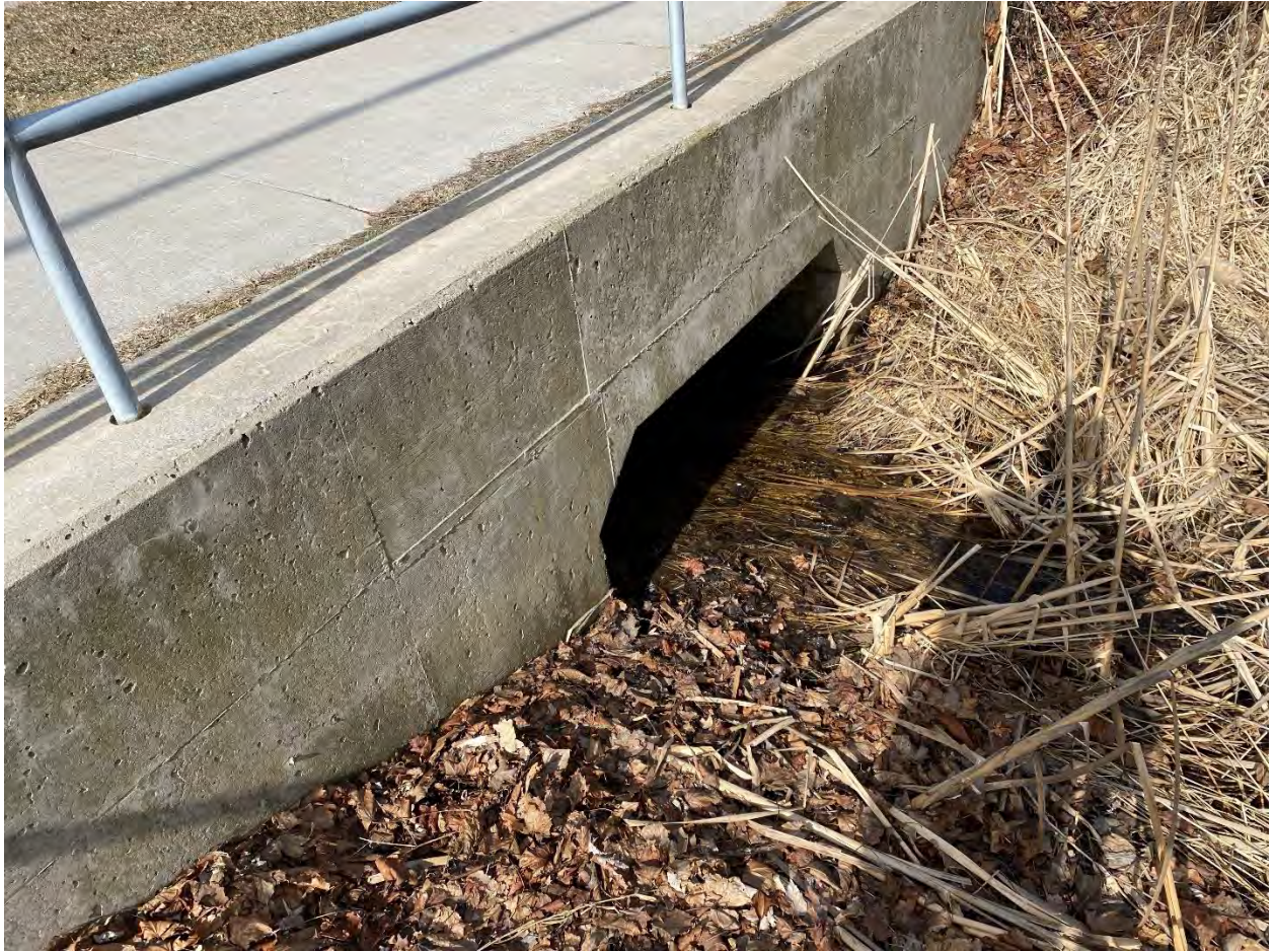
Trulls Road Culvert East Side (upstream inlet)
