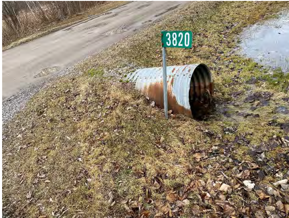
Sherry Lane Culvert South Side (downstream outlet)
