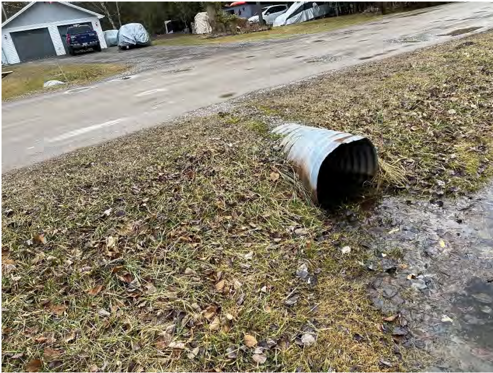
Sherry Lane Culvert North Side (upstream inlet)
