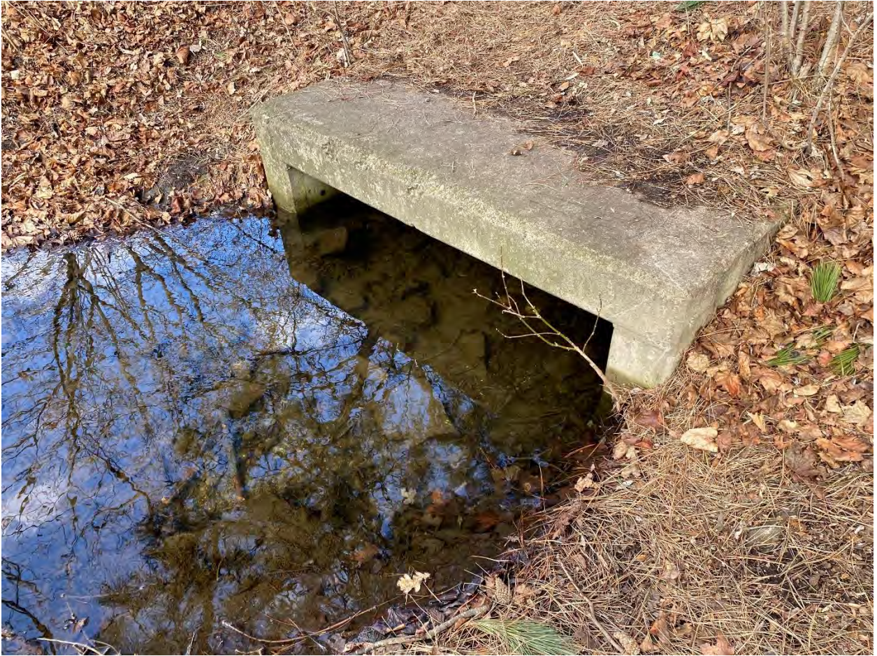
Devondale Street Culvert South Side (downstream outlet)
