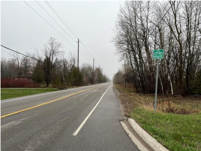
Plate 7: Looking north along Trulls Road (A.S.I., 2024)
