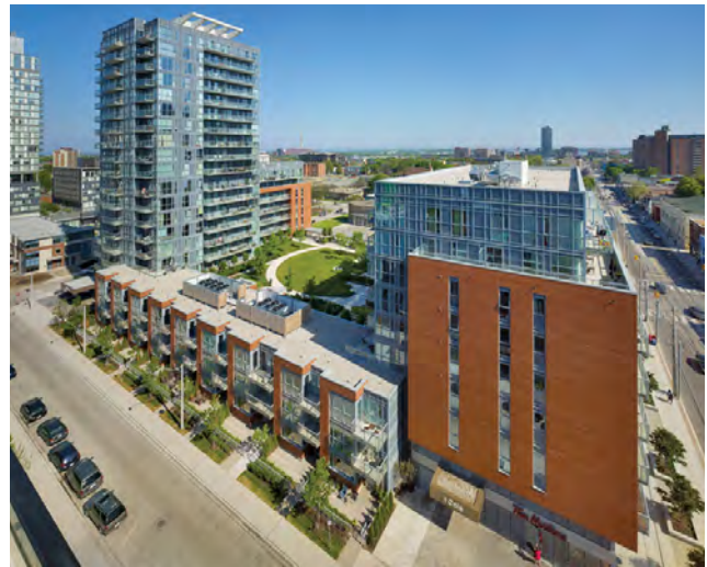
Figure 05: Buildings are sited to define street edges. The mid-rise building has retail at ground level and is located beside the sidewalk (right). The townhouse units have small front yard zones (left). A small setback (bottom) provides a public space at the building entrance and for retail spill-out.
