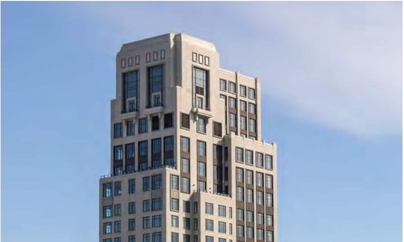
Figure 20: This mechanical penthouse is fully integrated with the architectural expression to create a dynamic skyline profile.
