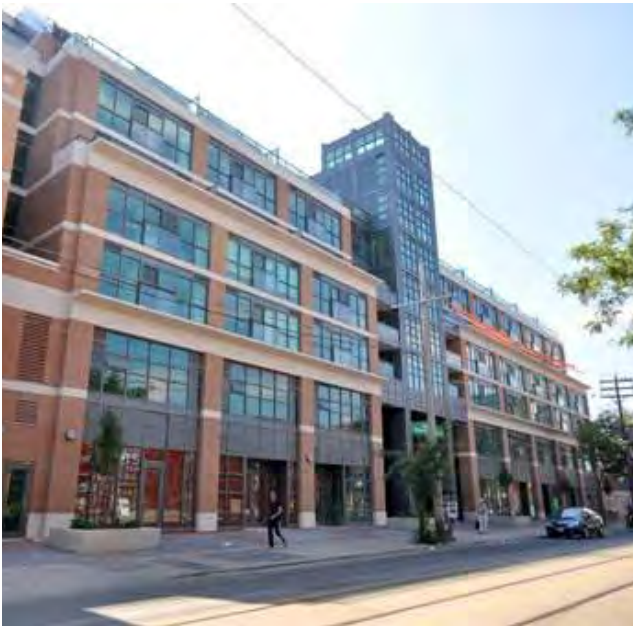
Figure 10: The main building entrance is emphasized through a central, taller massing element clad in an accent material. The entrance is a double height volume, and recessed for weather protection.
