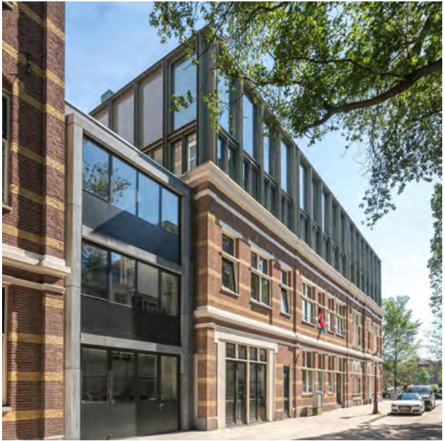
Figure 43: The heritage building reads as a distinct expression while being framed by new development that has similar massing and articulation.
