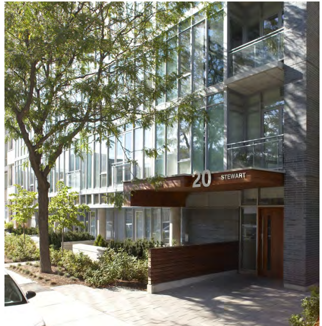
Figure 11: The building entrance is covered, with a small forecourt. The architectural expression above (balconies, brick) changes.
