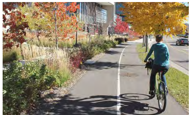
Figure 40: Multi-use paths along rights-of-way should be separated from vehicular travel lanes, for example, by planting buffer and grade shifts.
