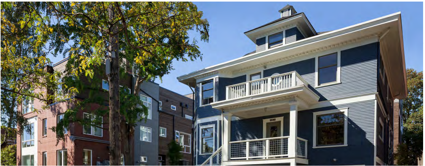
Figure 56: This infill project preserves a single detached house while intensifying with row housing that has a compatible scale and character with the existing streetscape.
