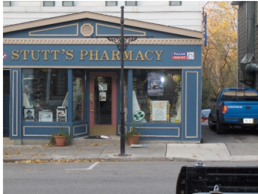
New poles on west side of Main Street. *Amended by 2017 Review
